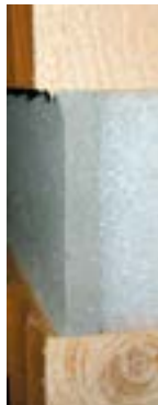
Replace plastic liner over the surface of the sealant
